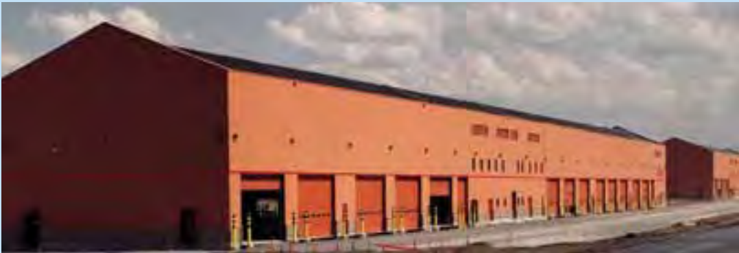
Saline County Public Library · Benton, AR Watchtower Educational Center · Patterson, NY Fort Drum Military Base · Fort Drum, NY
